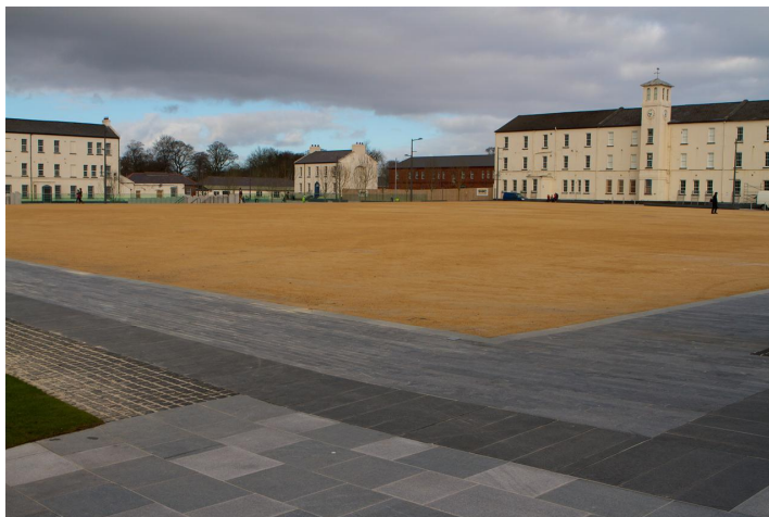
3. Feature Parade Ground Edging Detail : Define square by stone paving/ brick edge
